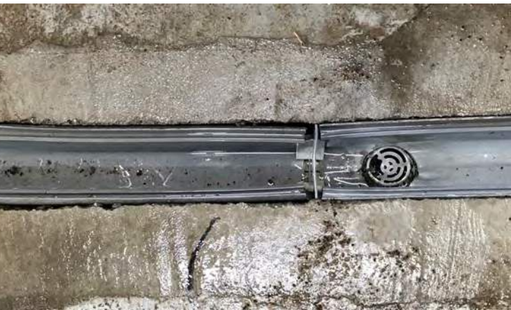
Plastic trench drain after one year of exposure to hot water in a brewery.
