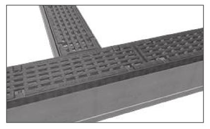
Attach grating and visually inspect the new joint for level appearance. Continue with installation of trench sections and preparation for concrete slab pour.
