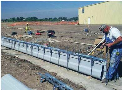
The 3000 Series™ high capacity drain system was recently installed between an airplane hangar and a taxiway at Salem Airport in Salem, Oregon. There was 360 feet of 3000 Series™ drain system put in place.
