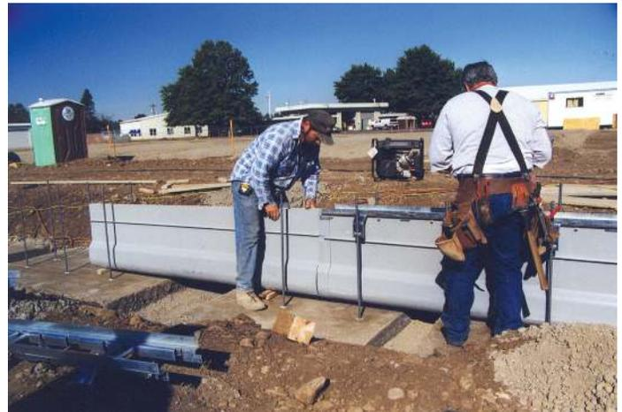
Taxiways must have a drainage system that can quickly move large amounts of water from the surface. With a flow capacity of up to 3000 gallons per minute, 3000 Series™ fit the bill perfectly. In fact, W.H. Pacific, the engineering firm for the project, chose 3000 Series™ over a competing drainage system because of its greater drainage capacity and ease of installation.
