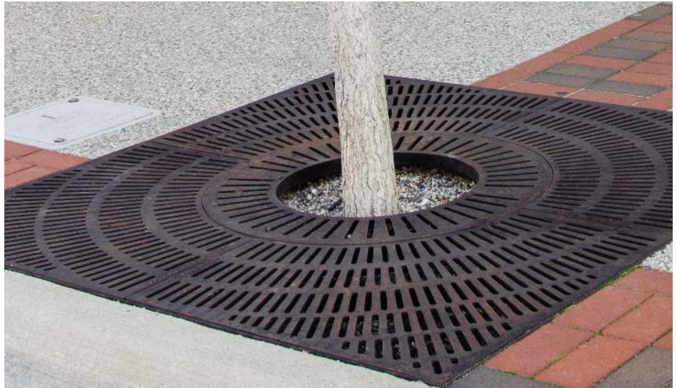
Center rings can be removed later to accommodate for tree growth.
