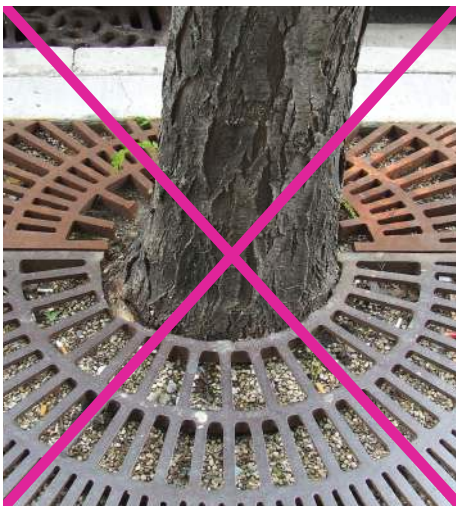
Poor size selection for the tree opening results in an unfinished look, significantly crowds the tree, and impairs proper tree growth.
